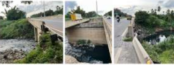
Existing condition of the river crossing the corridor
