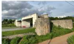
Existing condition of the unused overpass
